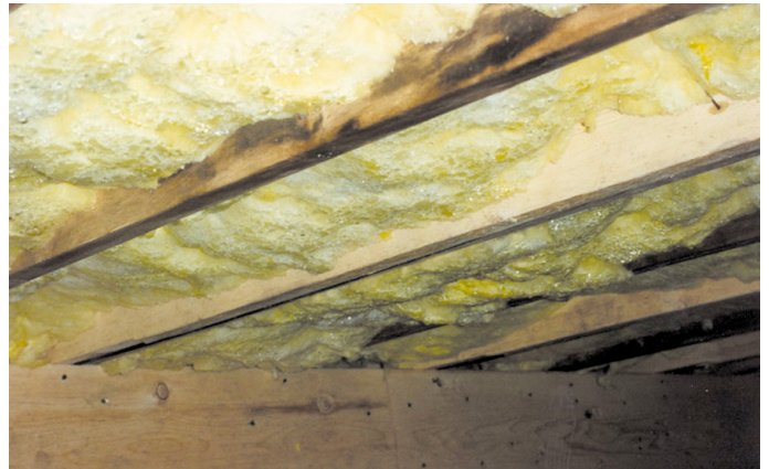
Photograph 1: Icky Crawlspace —Note the condensation on the underside of the fiberglass insulation and the rot at the exposed portions of the crawlspace floor joists.
