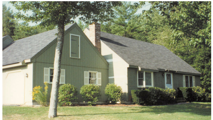
Photograph 2: Nice House Over Icky Crawlspace —This house with the crawlspace problem is in Washington, DC
