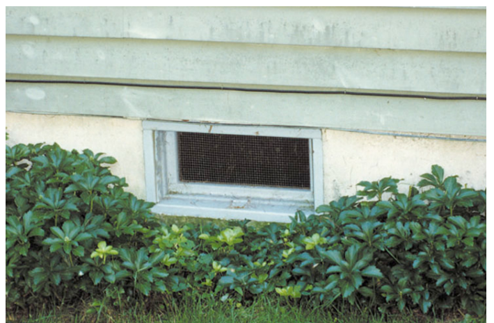
Photograph 3: Ventilation Opening —Crawlspace has plenty of cross ventilation and good drainage.
