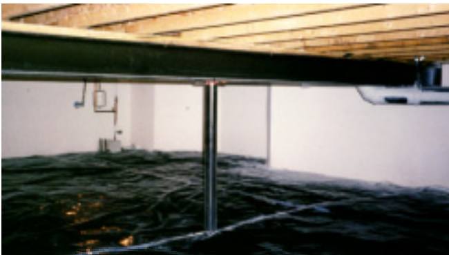
Photograph 5: Conditioned Crawlspace —The way all crawlspaces should look. Dry, warm, part of the house, not part of the outside or part of the ground. Insulated on the perimeter not in the floor. Beautiful.
